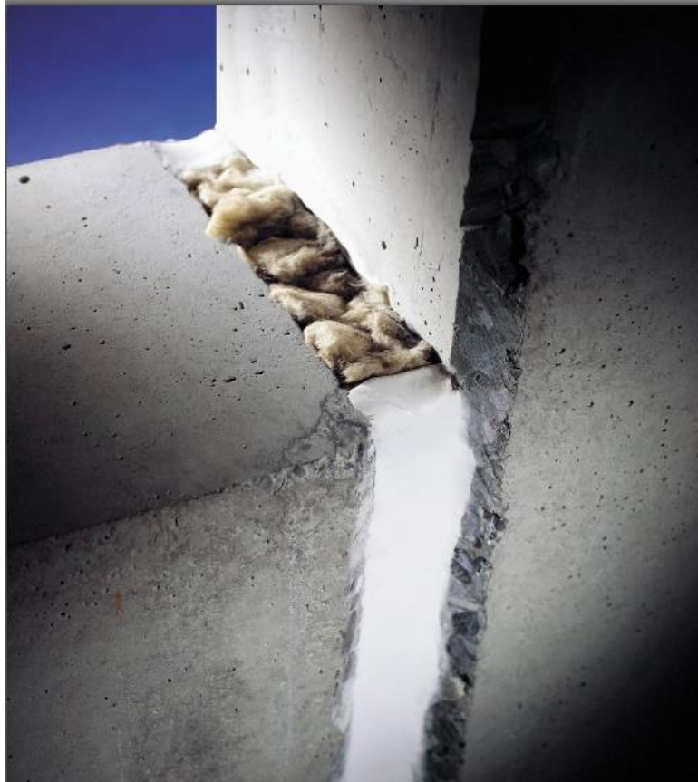
Figure 8: Sealant used for a fire resisting linear joint seal
