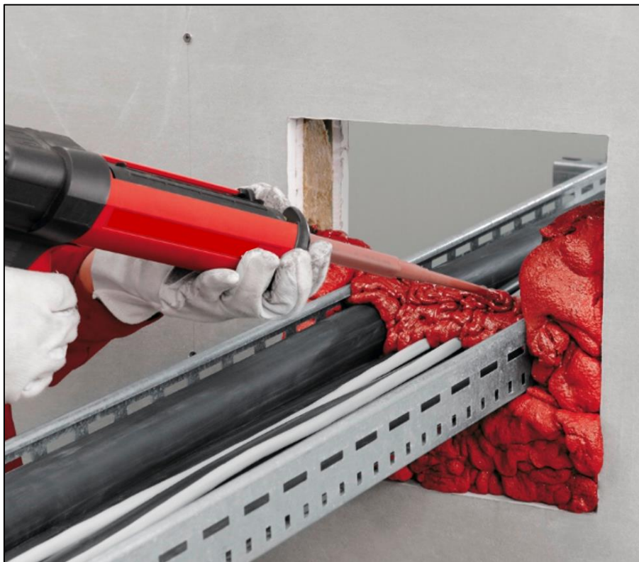
Figure 31: 2-component Polyurethane fire-stop foams correctly used for penetration seals
