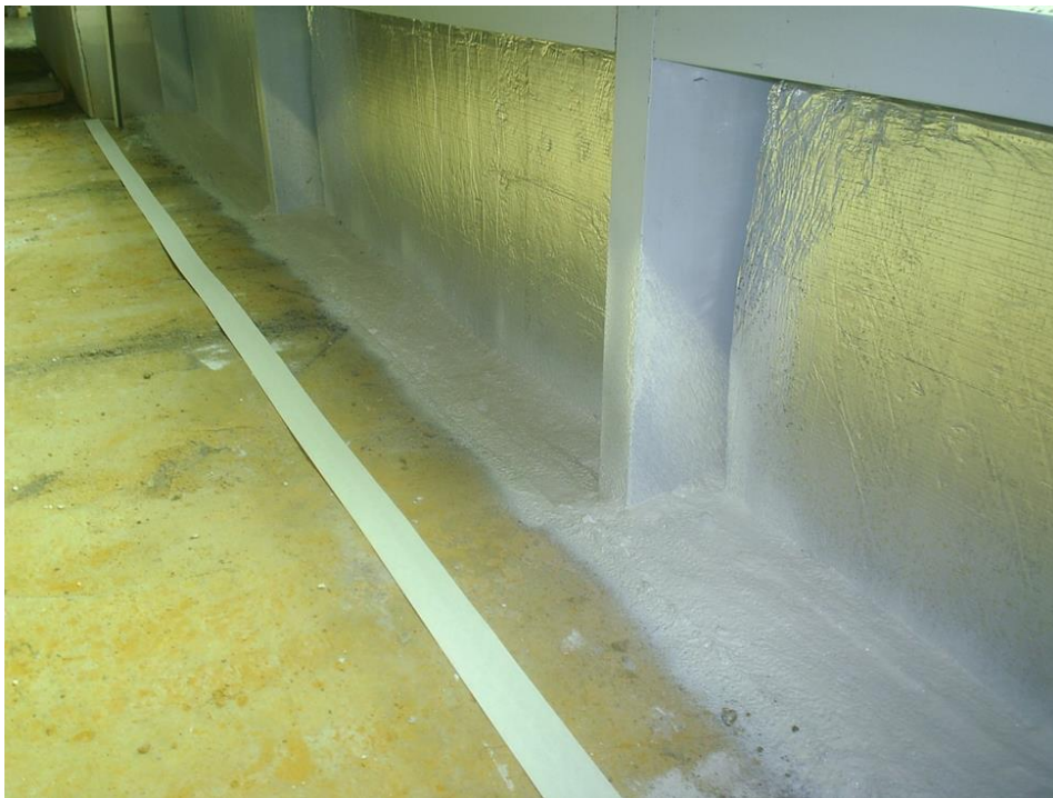
Figure 29 – Sprayed linear fire seal as fire-stopping to slab perimeter
