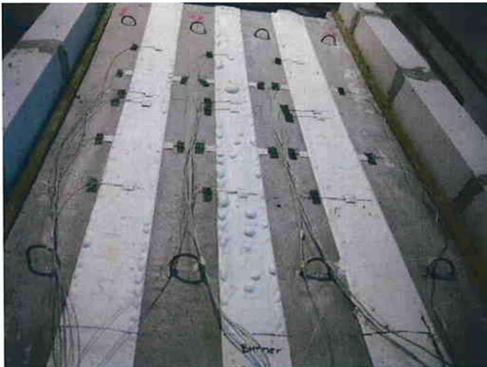
Figure 44: Linear joint seal installed for fire testing
