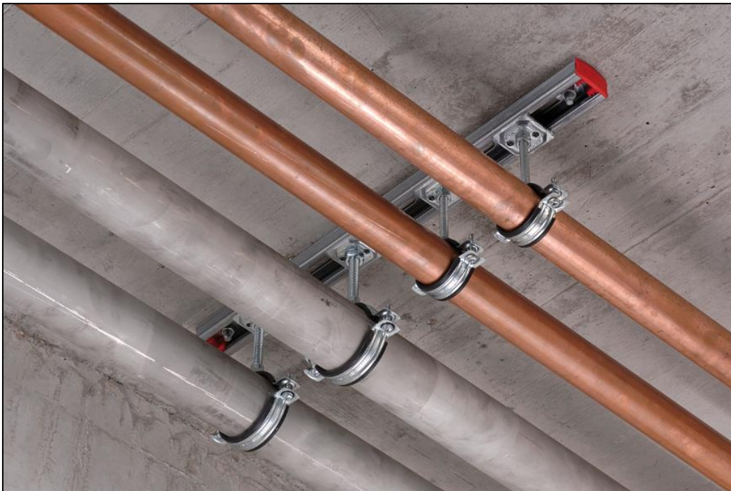
Figure 39: Example of fire rated service supports
