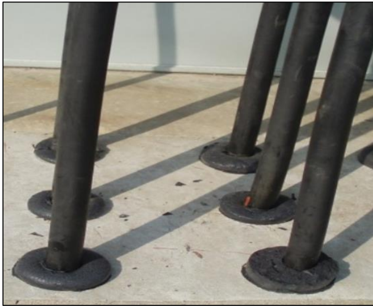
Figure 32: Silicone fire-stop foams correctly used for penetration seals
