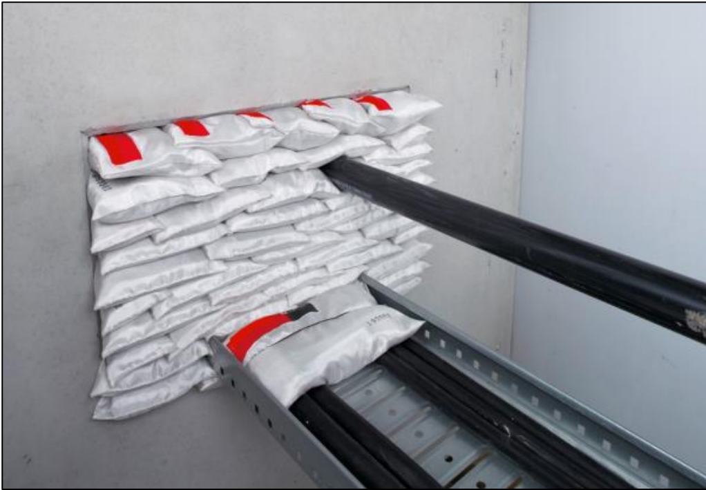
Figure 14: Pillows used to provide temporary fire-stopping of a horizontal cable tray
