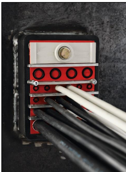
Figure 33 Examples of firestopping cable sleeve and transit
