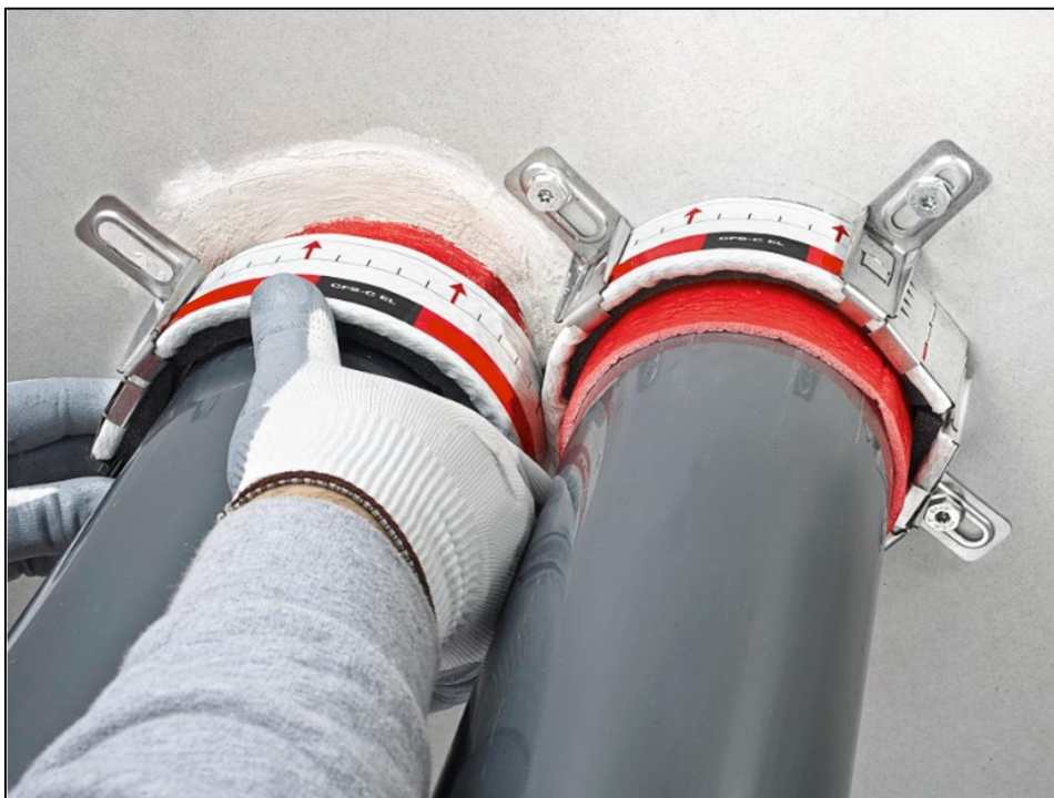
Figure 16: Pipe closure used around plastic pipes passing through a wall
