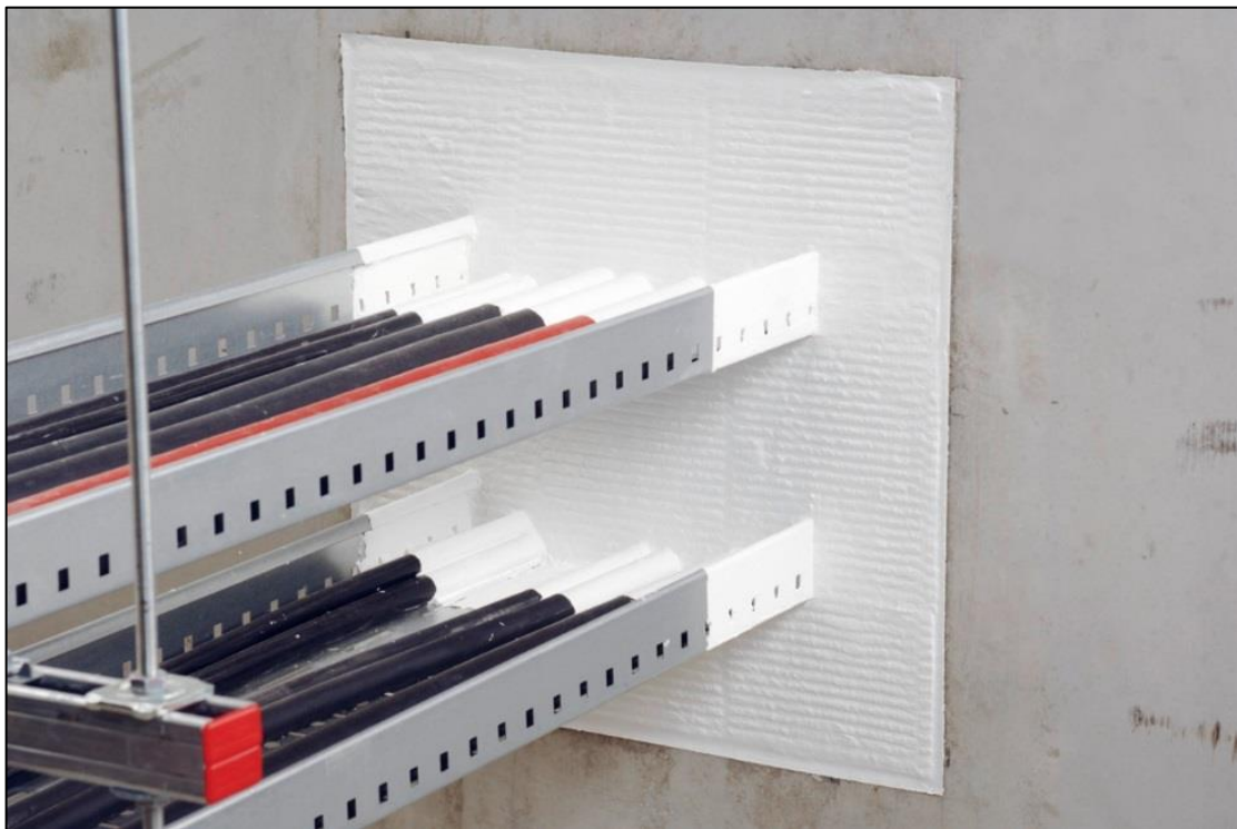
Figure 4: Coated batt used for a vertical penetration seal
