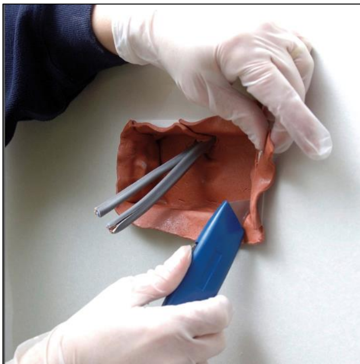
Figure 35: Intumescent putty pad to fire-stop electrical outlet – being installed
