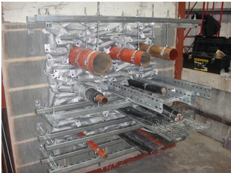
Figure 42: Pillow penetration seal installed for fire testing
