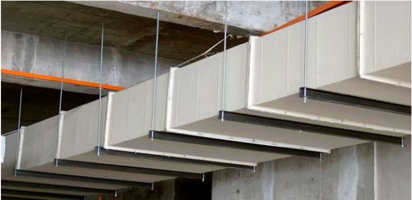
Fire resisting ductwork being installed
