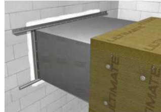
Step 4a: Reinforcing a rectangular duct
