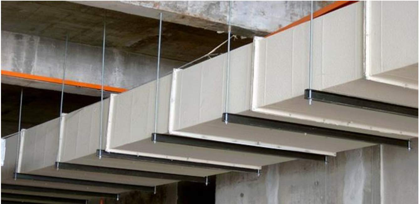
Fire resisting ductwork being installed
